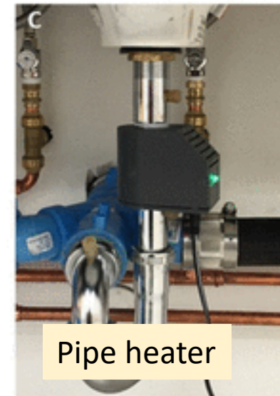
Figure 1. Tuba Drain assembled out of standard copper parts joined to standard plumbing.
